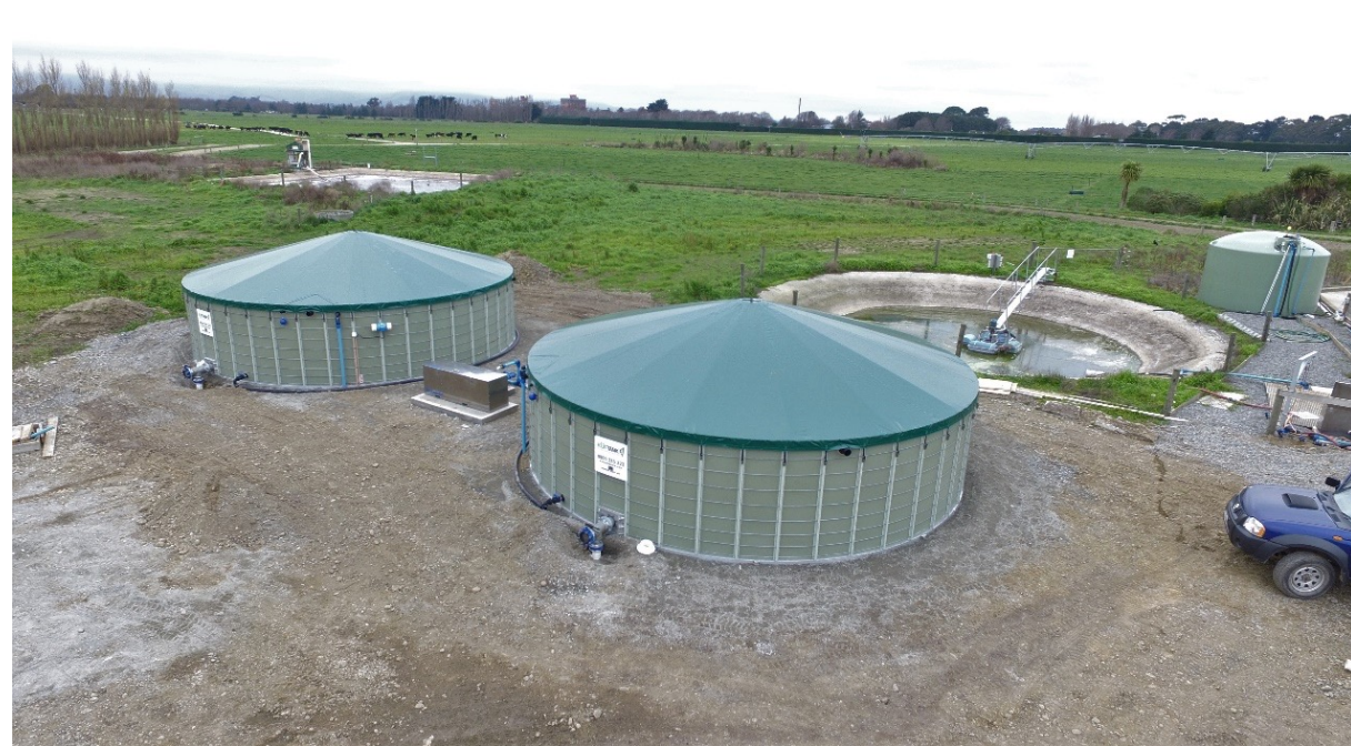
100,000 L effluent tanks (with gas capture facilities)
